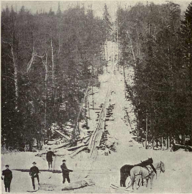
Fig 1. A Log Chute, Canada.
